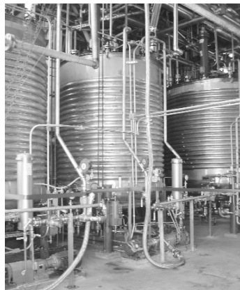
◀ A final view of the storage tanks after installation.
