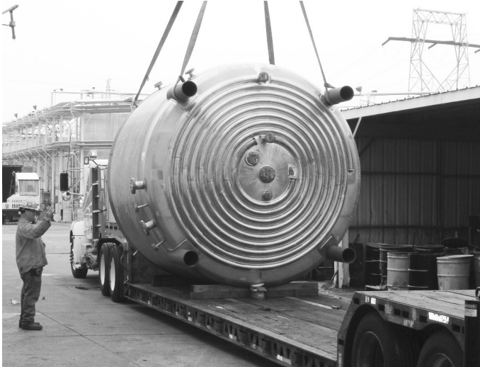
▲ Clay Buxton unloads one of the storage tanks at the Elantas, PDG site.
